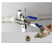
Let the PE pipe go through the Nut, then connect the PE pipe with the Water Inlet Valve, and rotate the Nut tightly.
