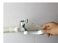
Tape the Water Outlet Faucet with Teflon
