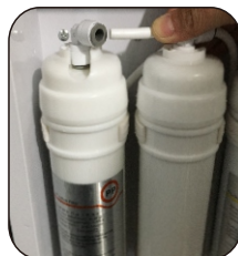
Disconnect the Blue Locker Press the Ring in the Joint, and stretch the PE pipe
