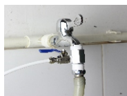
Connect the Water Inlet Valve with the Faucet, and connect the original pipe with the Three-way joint.
