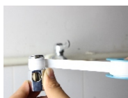
Tape the Three-way Joint with Teflon
