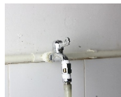
Connect the Three-way Joint with the Water Outlet Tightly
